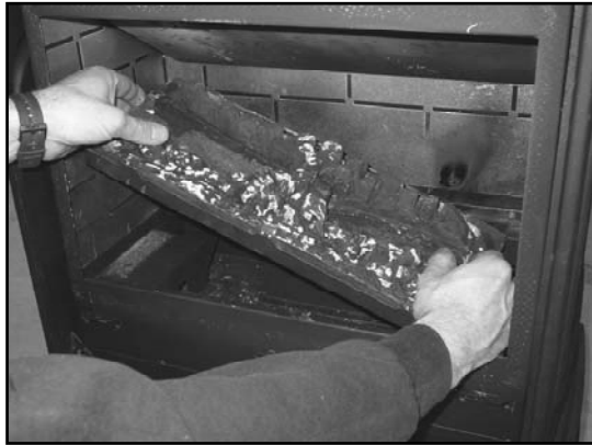
Figure 8.9 Remove burner by sliding the shutter to the right, lifting up the left side of the burner and sliding it the the left.
