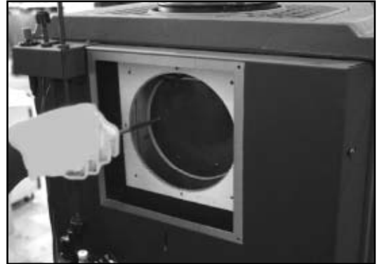
Figure 8.2 Remove the rear outer flue cover plate (with the damper adjustment plate attached). Ensure that the gaskets and grommets stay in place.
