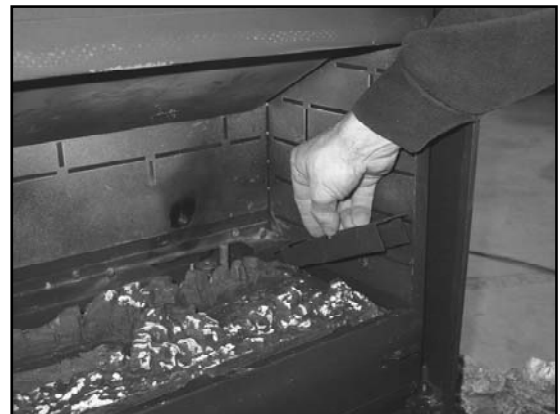
Figure 8.8 To remove the burner pan locators from the left and right sides of the burner, remove one screw from each side, lift locators up and out.
