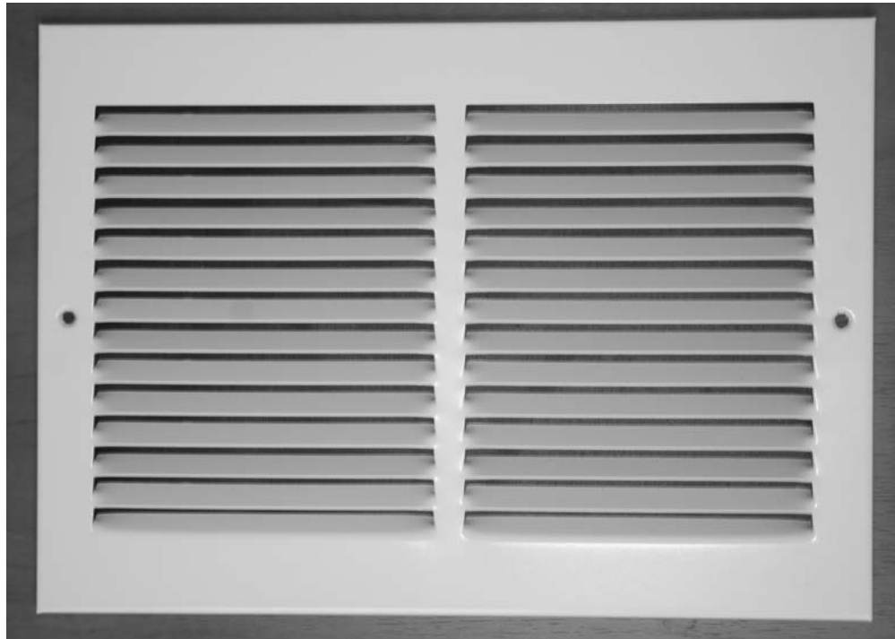
Figure 7: Finished installation with register
