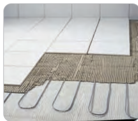
Typical undertile installation
