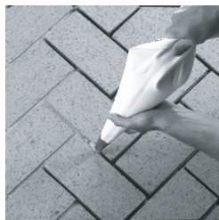
Figure 23 - Grouting Brick
