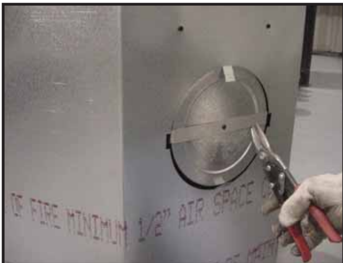
Figure 9.7 Cut the metal retaining band and fold the sides out.
