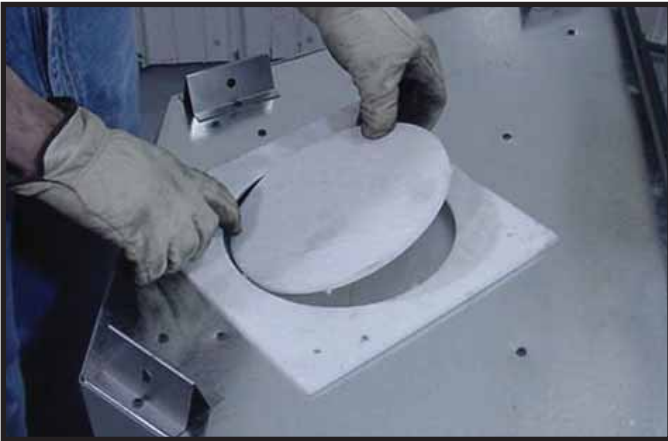
Figure 9.2 Remove the center insulation plug.
