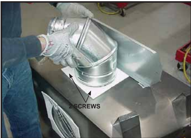
Figure 7.7 To attach the first section of vent pipe, make sure to use the fiberglass gasket to seal between the first vent component and the outer fireplace wrap. Use 2 self tapping screws to secure the gasket to the outer wrap.
