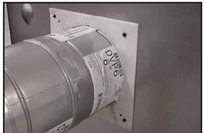
Figure 7.12 Attach the first vent section (it will snap into place). Slide the insulation gasket onto the vent section, up against the appliance and over the tabs. Use two self-tapping screws to secure gasket to outer wrap.
