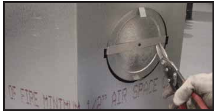
Figure 7.9 Cut the metal retaining band and fold the sides out.
