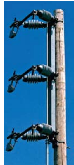
Phase-over-Phase Mounting
