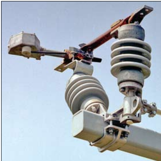
Chance 15.5, 27 and 38 kV Duogap expulsion interrupters .
